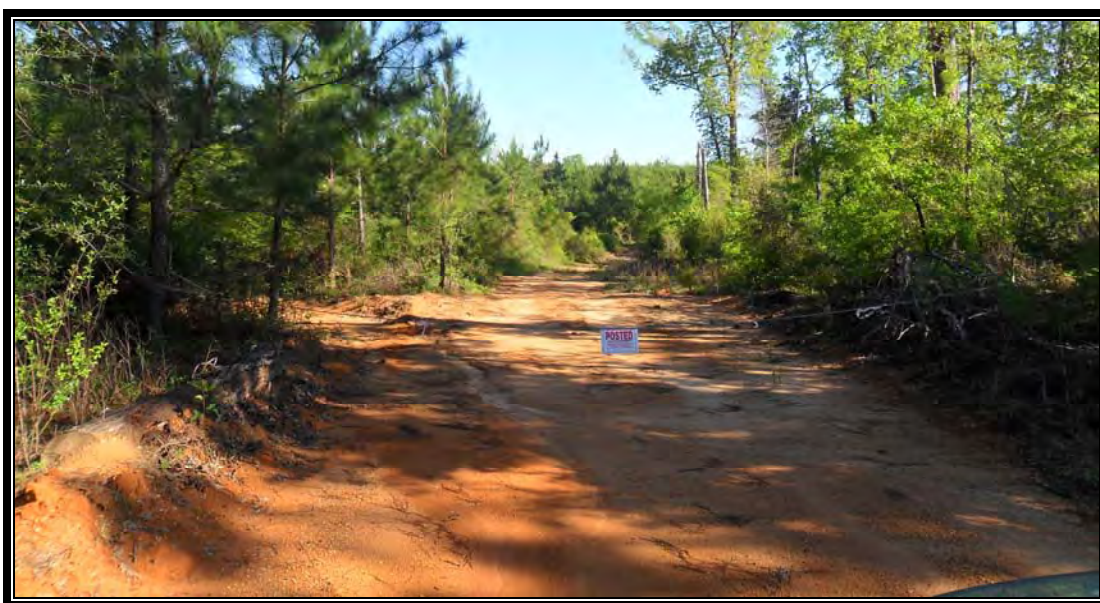
View of Entrance into Comp #6 from Bratt Road – taken 4/12/2011
